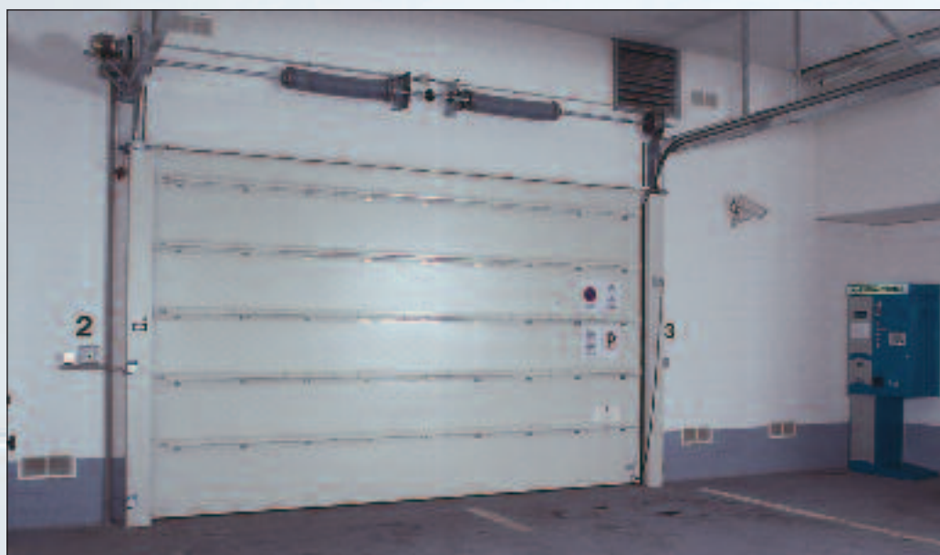
T30 Sectionaltor in Tiefgarage.
